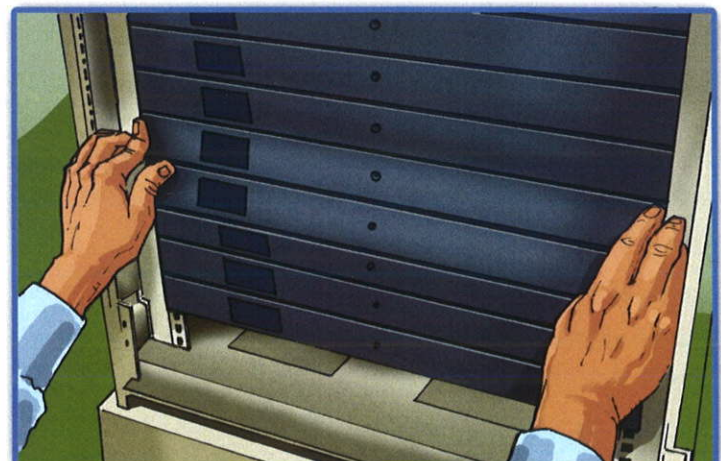
Insert the desired size of panel to fit the open rack space available
